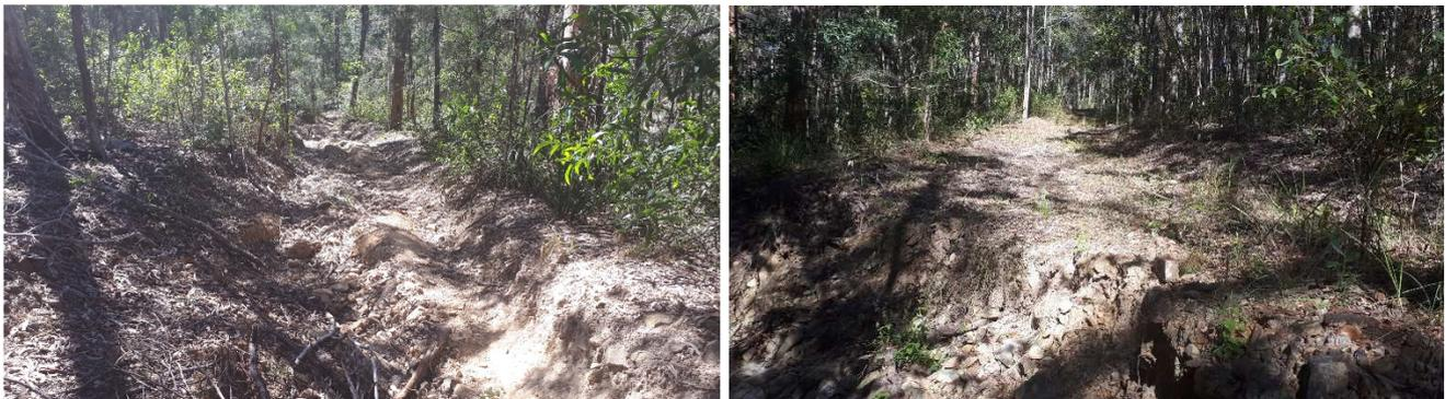
Images of track washouts preventing vehicle access for site management through ACR Year 1.
