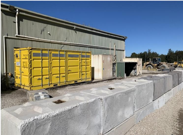
Figure 4 – Self-bunded enclosed chemical storage
