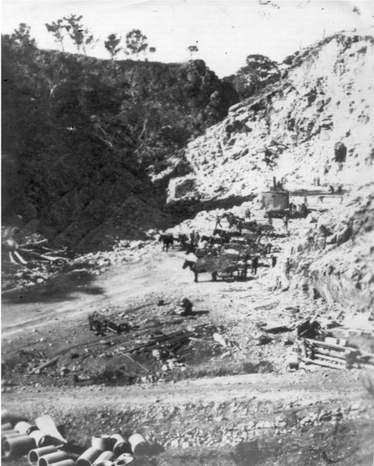
Plate 2.11 Marulan South Limestone Mine showing drays ready to transport limestone from the pit (courtesy of Boral Cement Limited)
