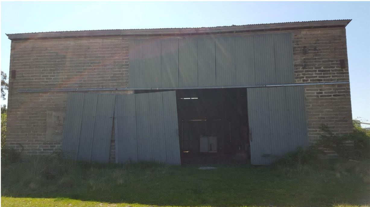
Plate 3.11 Front of the control room (MS04\_11), facing west, showing the corrugated iron rolling doors which would have opened to let out heat (at the base) and for the rope to rotate (top) (20151006\_144642).
