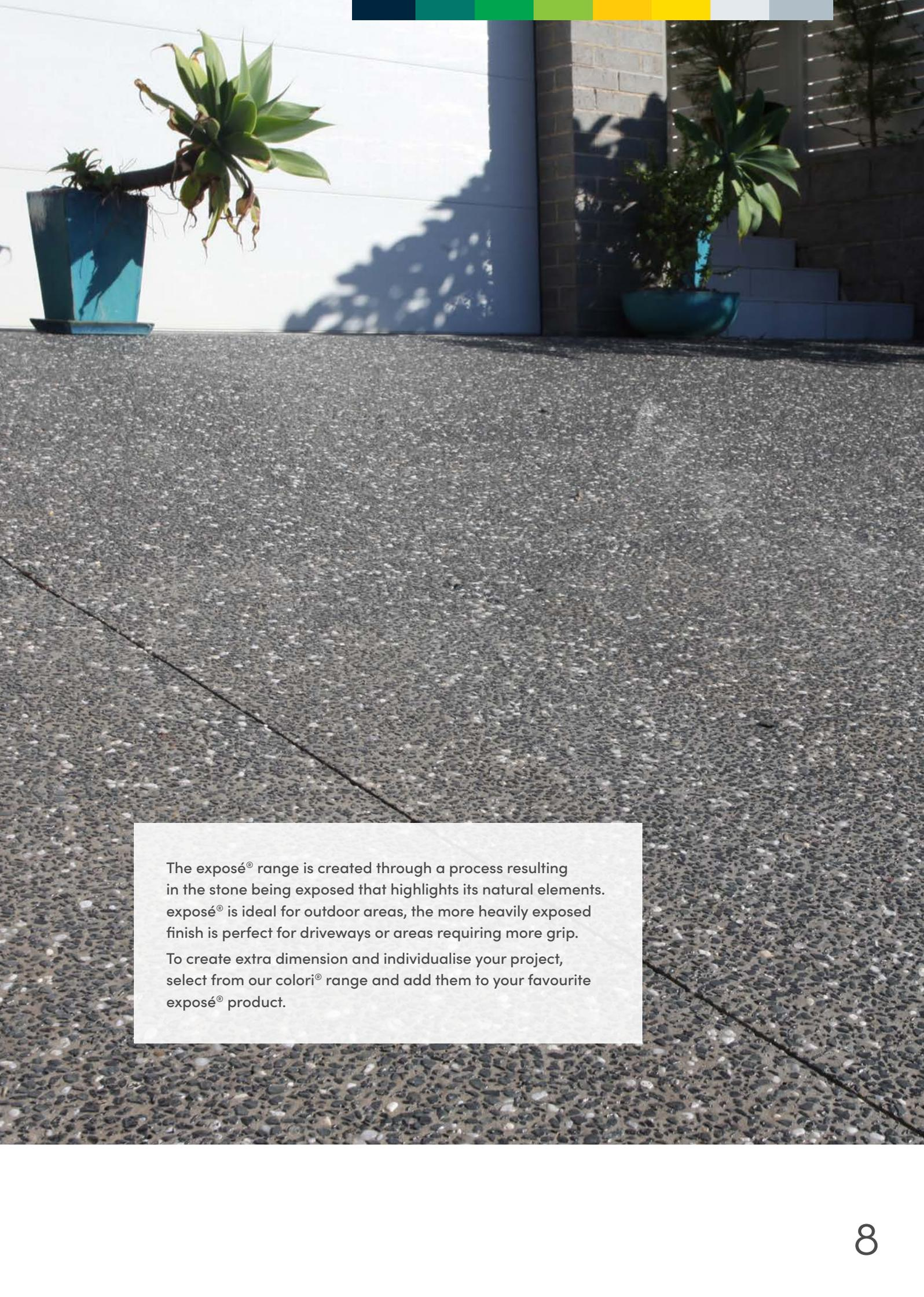
The exposé® range is created through a process resulting in the stone being exposed that highlights its natural elements. exposé® is ideal for outdoor areas, the more heavily exposed finish is perfect for driveways or areas requiring more grip.
